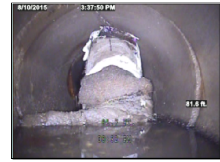
PICTURE 2 PIPE BLOCKAGE
